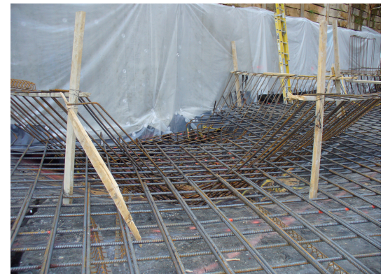
Figure 2: Mat Slab Reinforcement
